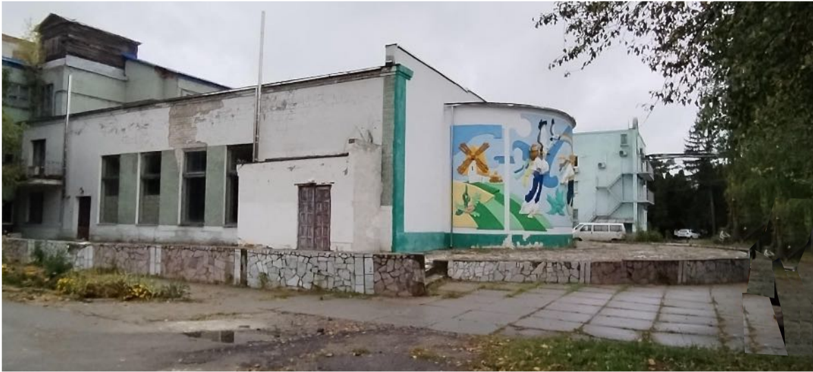
Existing condition. Photofixation
